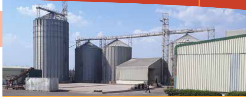
Milling Plant & Grain storage Silos
